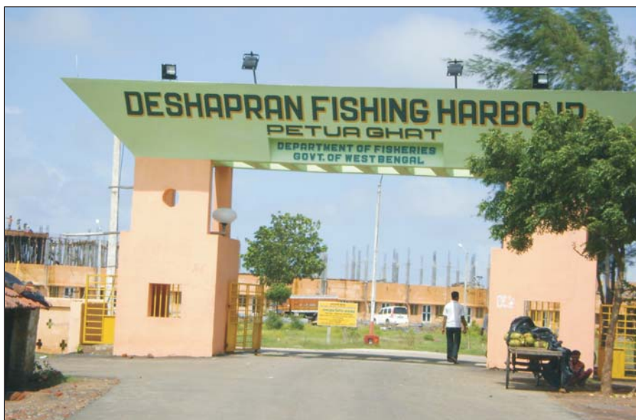
Deshapran fishing harbour under construction in West Bengal
