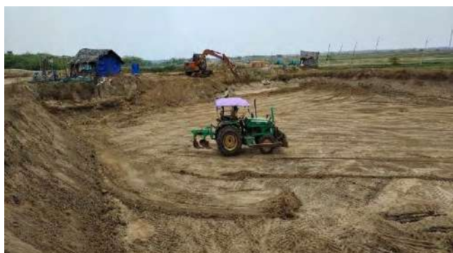
Fig. 5: Heightening the bunds
